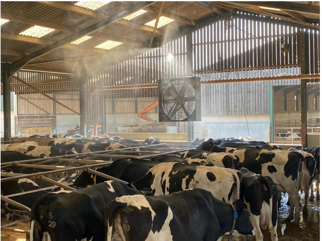
Picture 6 Example of a stable with a misting system [13]
